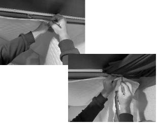
**NOTE**: Some trailer models will require relocating curtain rails and other hardware. Curtain rails usually move about 2 inches, this will not affect the function of your curtains. Remove the curtain rail, install your liners, then reinstall the the curtain next to the liners. Gear net pad eyes will also require relocation or replacement in a new location.
